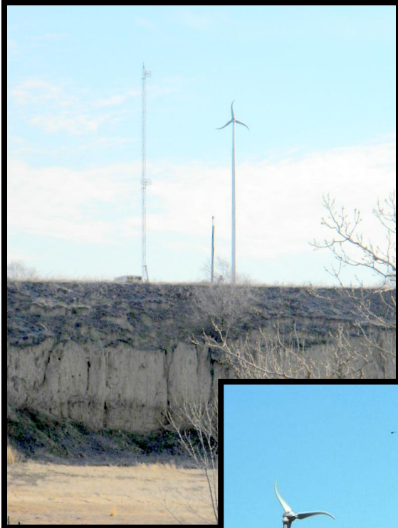
Net Metering Small Wind Energy System Rural Furnas County, Nebraska
