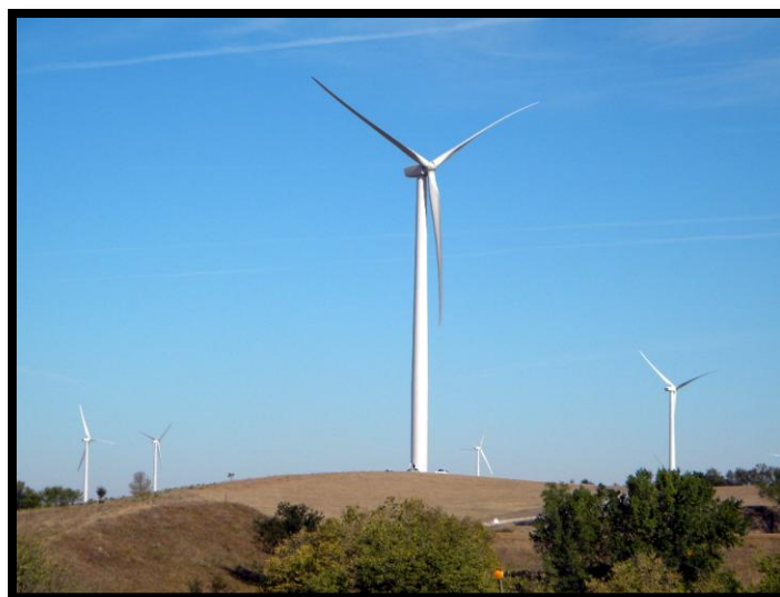
Broken Bow Nebraska Wind Facility
